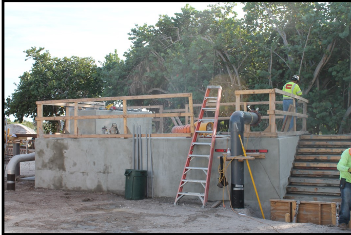
The new brine sump nearing completion
