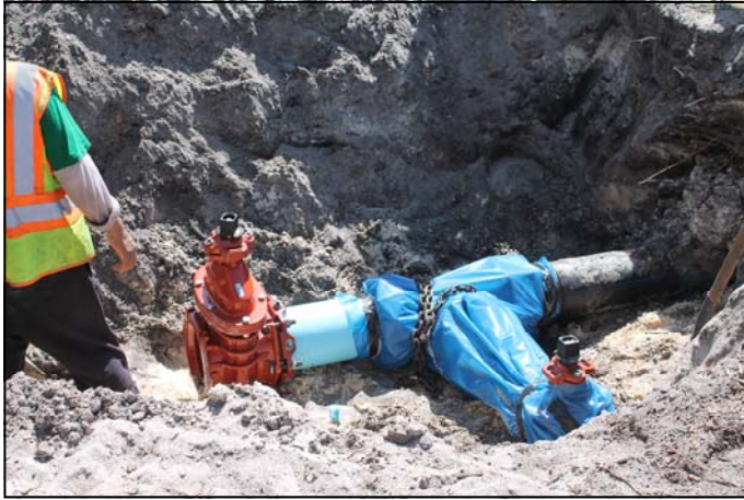
New Piping Being Installed in Sea Oats
