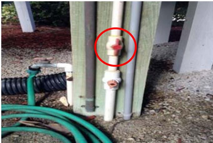
A Quarter Turn PVC Ball Valve in the On Position
