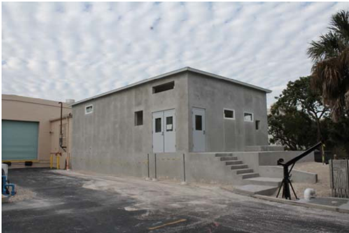
Southern View of Distribution Pump Station Addition
