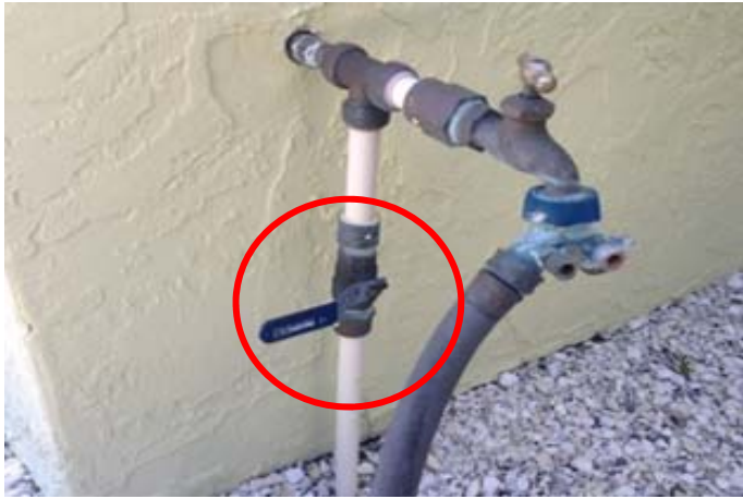
A Quarter Turn Single Lever Ball Valve in the Off Position
