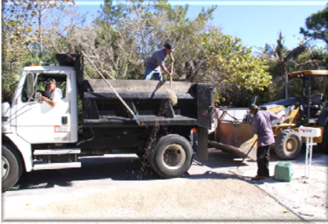
Driveway restoration in Sanibel Bayous
