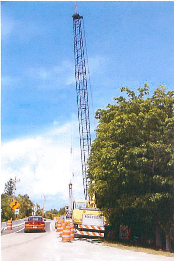
City of Sanibel culvert/bridge project
