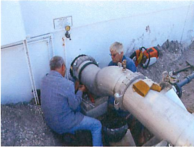
John, right, working on well line tie-in.
