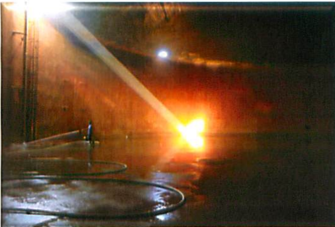
Cleaning & Inspecting a Five Million Gallon Storage Tank
