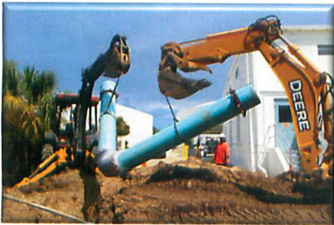
Installation of New Transfer Line
