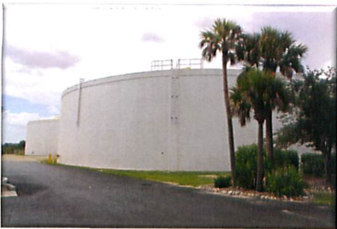
Twin Five Million Gallon Storage Tanks
