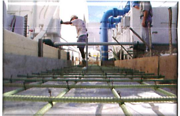
Concrete Pipe Support Pad
