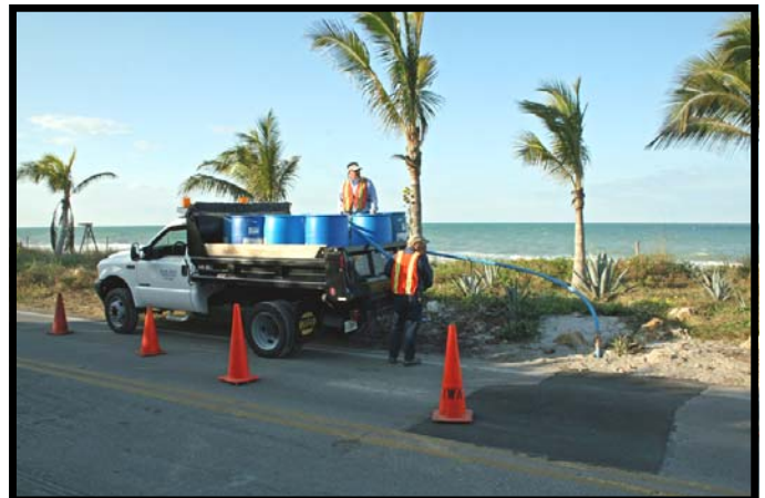
Manning the air vent during grouting
