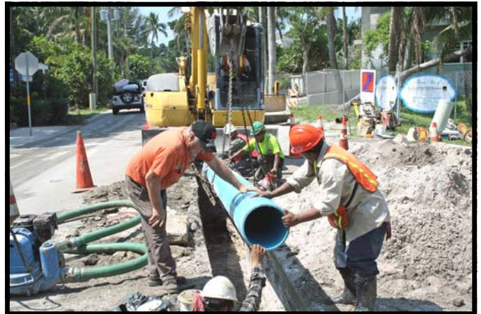
Setting a Stick of 12" Pipe in the Village
