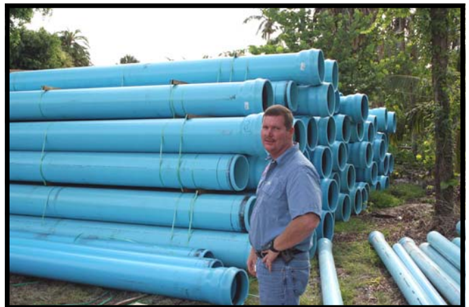
Distribution Manager Joe Scofield, Inspecting 16" Pipe
